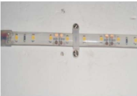
○ Installation is finished;
