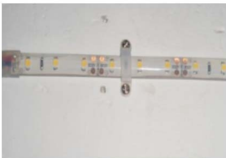
○ Installation is complete
