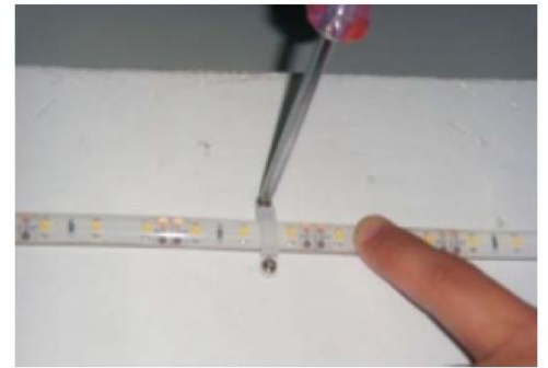
○ Mounted the snap spring.
